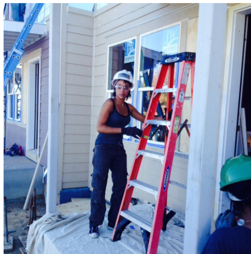
ULI Colorado volunteers help build Habitat for Humanity's first attached housing in Denver's Montbello neighborhood.
