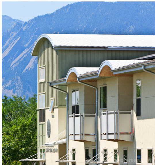
Boulder's Holiday Neighborhood is a 27-acre infill community blending everything from Habitat homes to deed-restricted middle-income to market rate townhomes in a walkable, transit-served setting.
